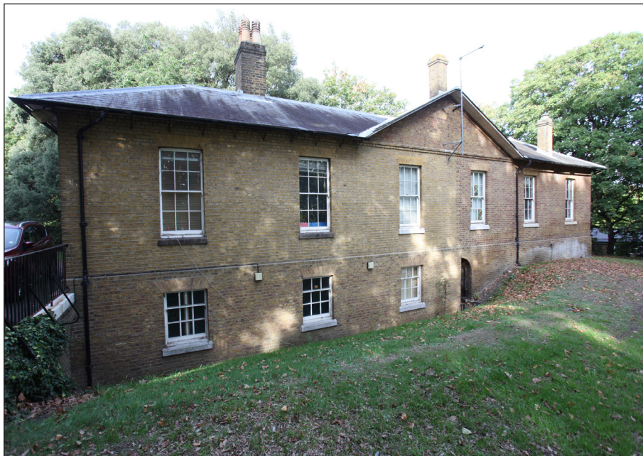
Plate 6) East facing elevation of the Observatory Married Quarters showing the contrast in brickwork resulting from the repairs to the structure
